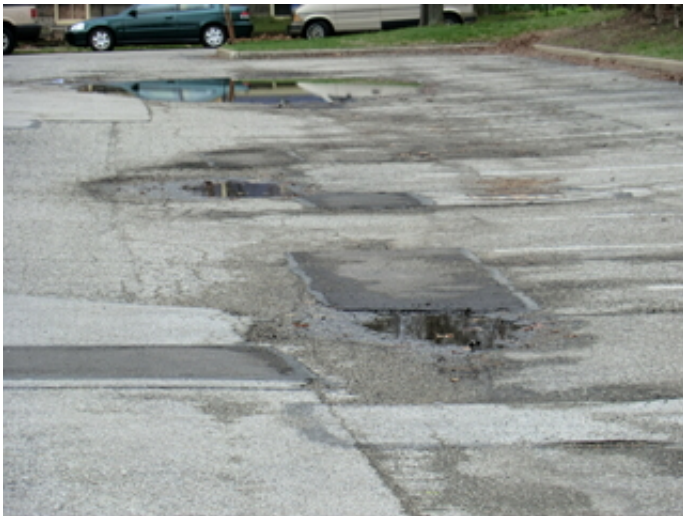
Deteriorated asphalt paving.
