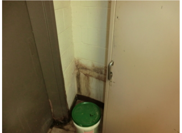
Evidence of water penetration.
