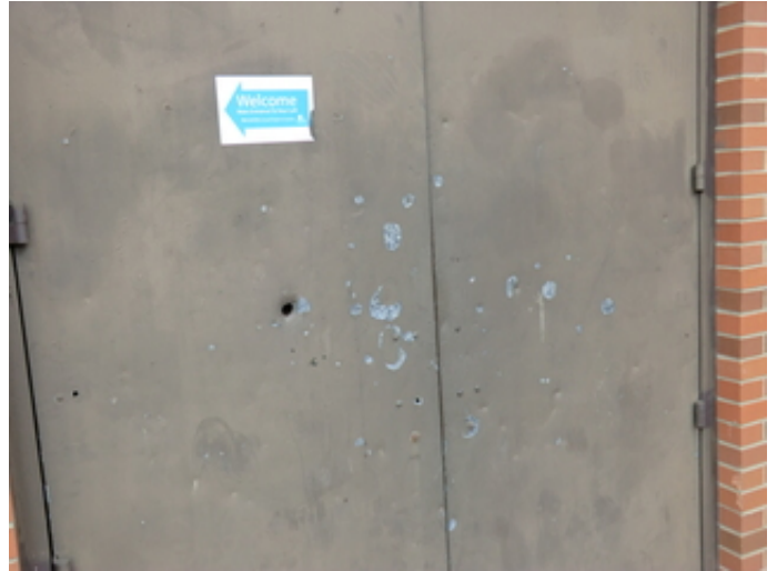
Damaged exit doors.
