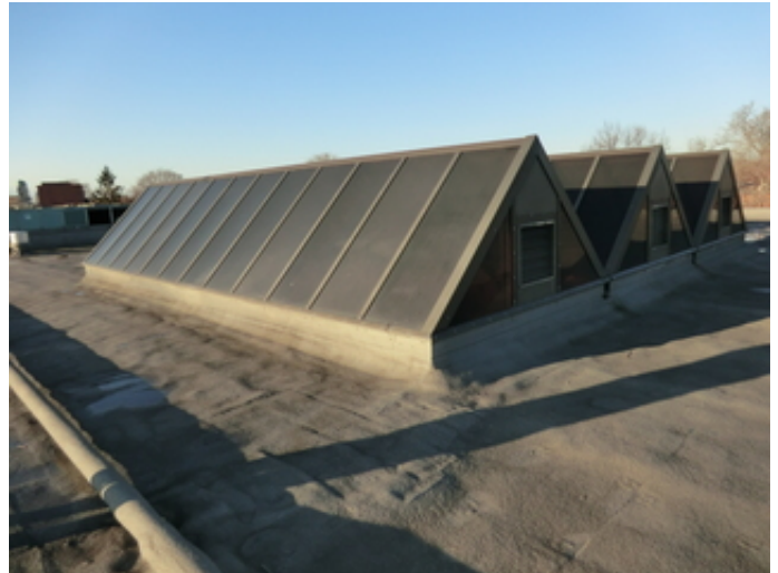
Skylights are vulnerable to water penetration.
