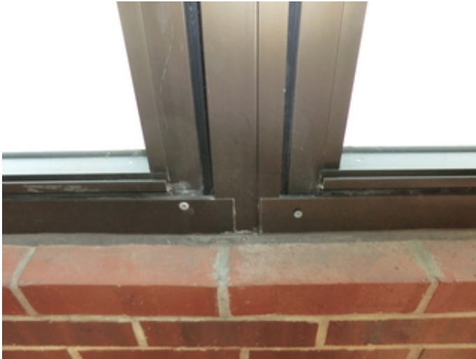
This window offers little to no thermal performance..
