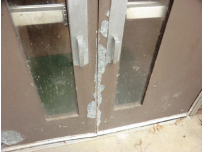
Misaligned corroding doors.
