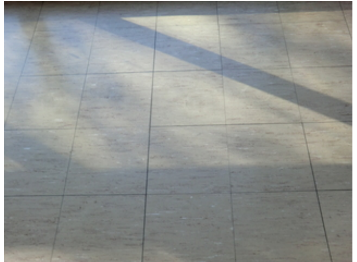
Floor tiles are separating at the joints.
