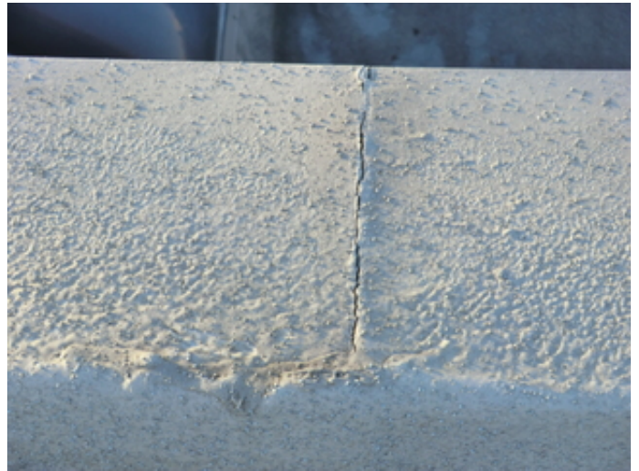
Roofing material cracked at coping joints.
