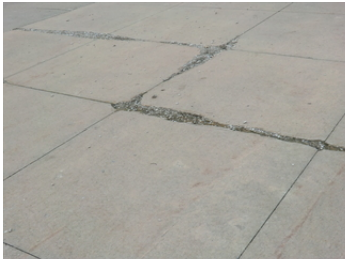
Deteriorated concrete paving.
