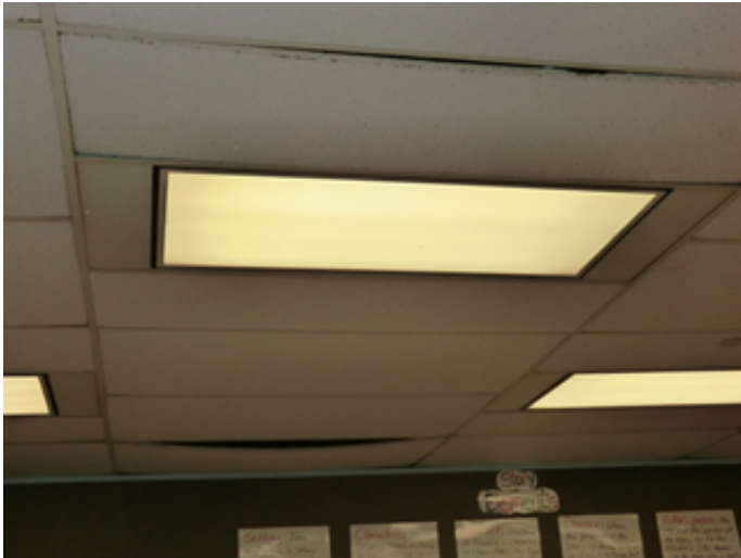
Ceiling tiles are sagging and falling away from the grid.
