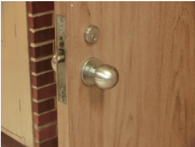
Door hardware is not ADA compliant.
