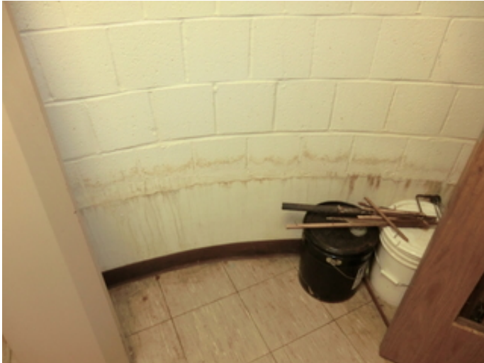
Evidence of water penetration
