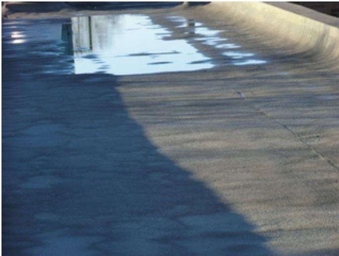
Large ponds observed on the roof.
