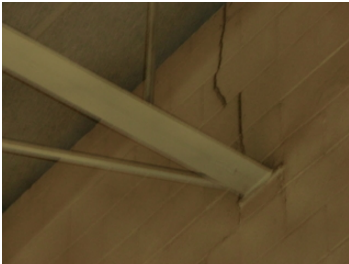
Cracks in wall above joist bearing.
