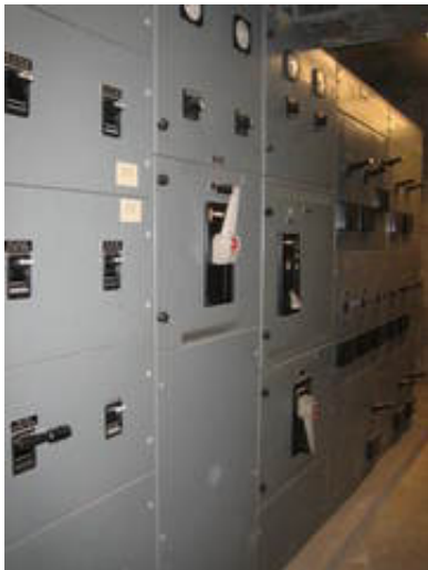
Main distribution panel
