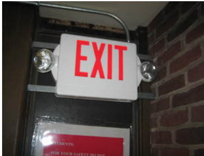
Corridor mounted emergency/exit fixture
