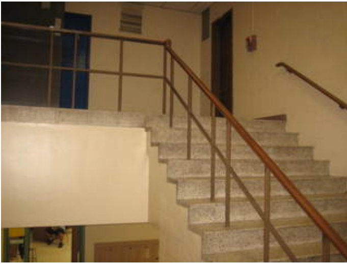
Open non-compliant stair
