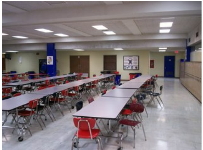
Lighting in student dining area
