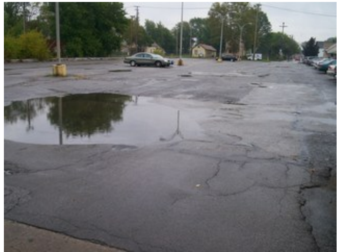
Ponding in asphalt parking lot in poor condition
