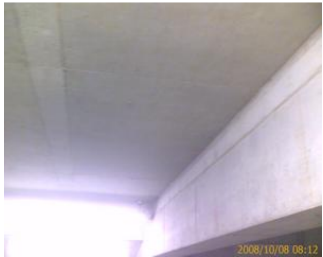
Typical cast-in-place concrete intermediate floor
