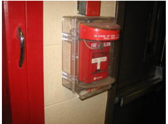
Corridor mounted fire alarm pull station
