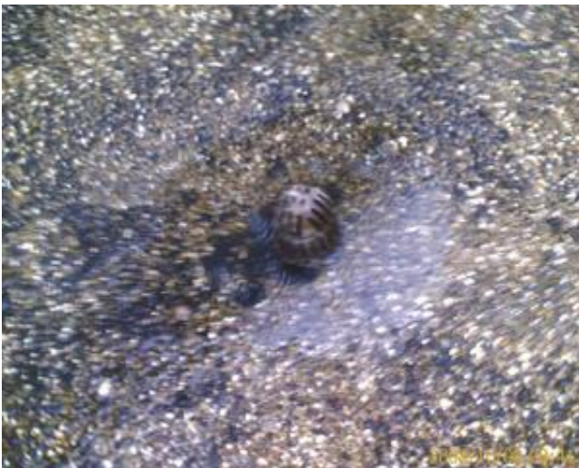
Typical roof drain condition
