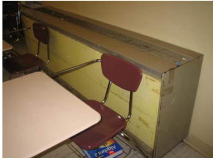
1970 Classroom unit ventilator
