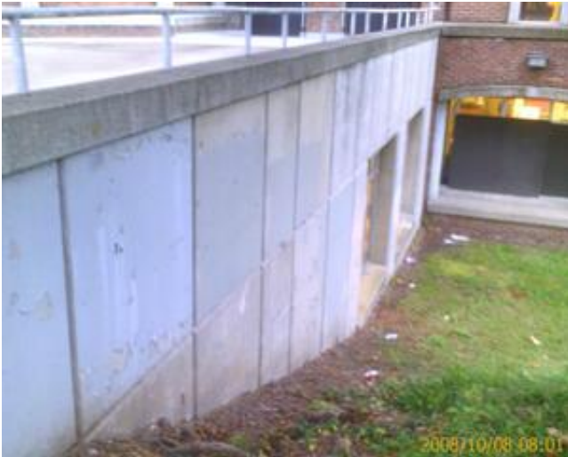
Typical cast-in-place concrete retention wall
