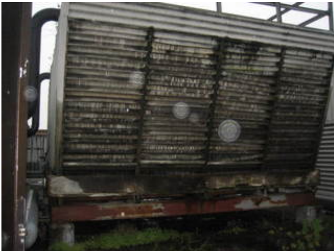
Rooftop mounted chiller
