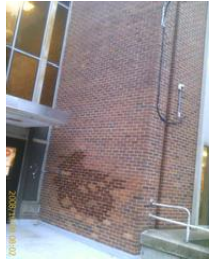
Typical exterior masonry condition
