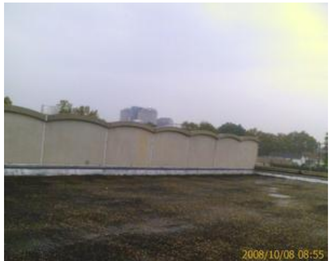
Typical roofing condition
