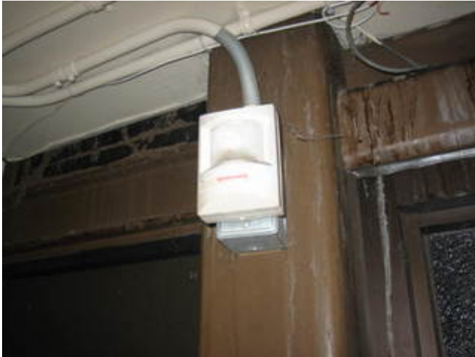
Corridor mounted motion sensor
