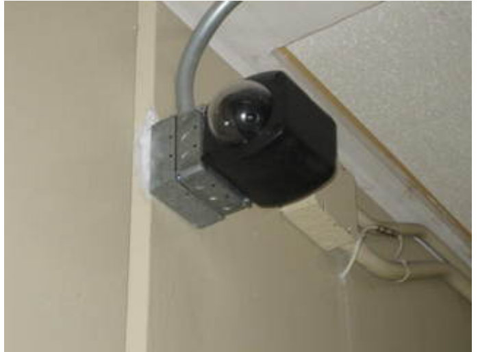
Corridor mounted security camera
