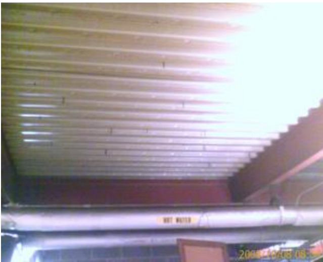
Typical metal deck roof structure
