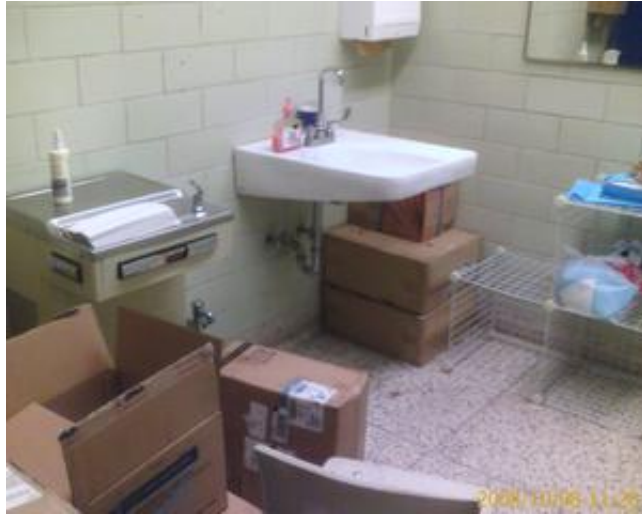
Typical ADA complainant lavatory sink
