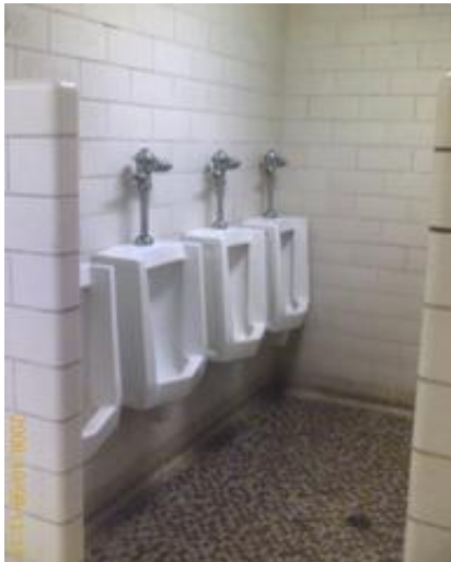
Typical urinal condition
