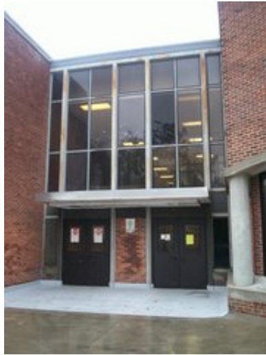
Exterior entrance doors
