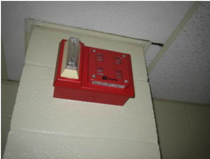
Corridor mounted horn/strobe device
