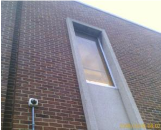
Typical lintel condition
