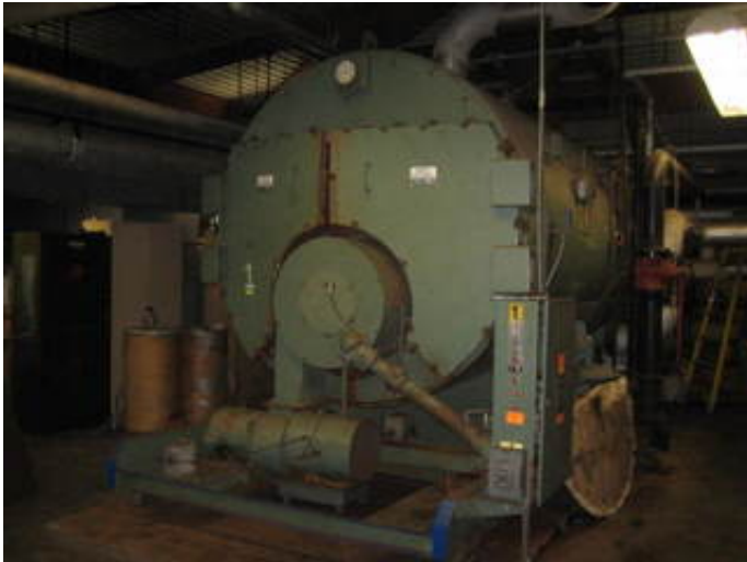
Natural gas fired boilers
