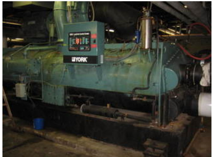
Cold water exchanger
