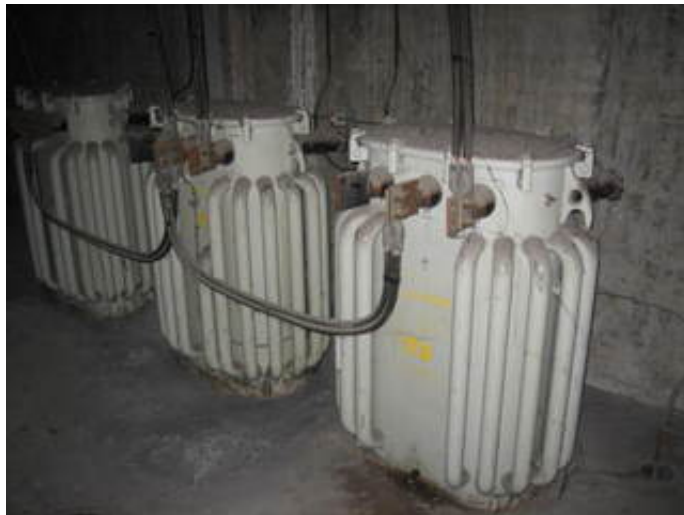
Vault / pad mounted transformers
