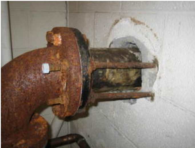
Water service entry
