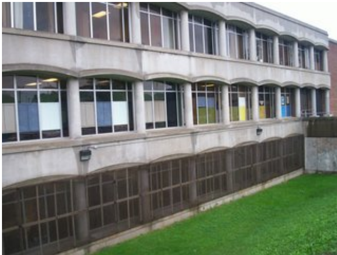
Windows at classrooms
