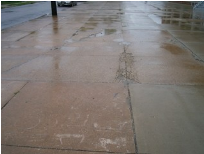
Concrete sidewalk in deteriorating condition
