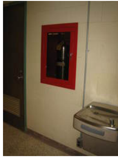
Corridor mounted fire extinguisher cabinet
