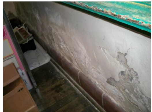
Damaged plaster
