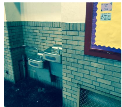
High / Low electric water coolers
