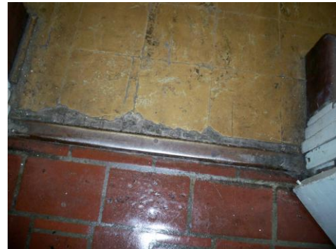
Damaged VAT flooring
