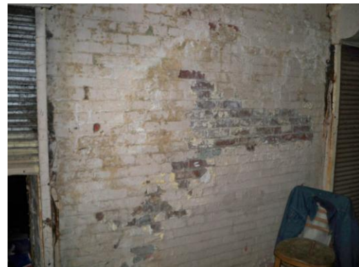
Interior brick wall in basement
