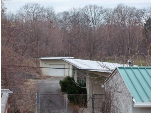
Greenhouse Roof (center bldg)
