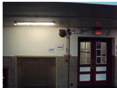
Non-compliant exit sign
