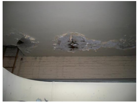
Plaster damage in ceiling
