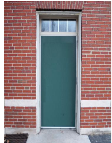
Typical exterior door
