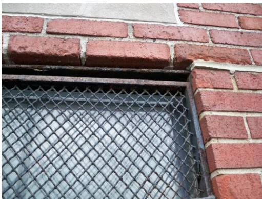
Delaminating Lintels at Boiler House
