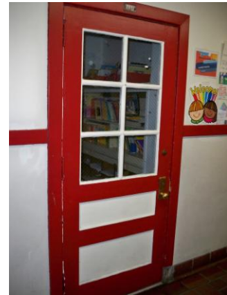
Old wood doors without ADA hardware
