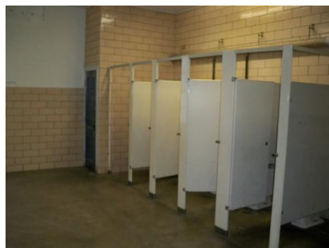
Non-ADA toilet partitions
