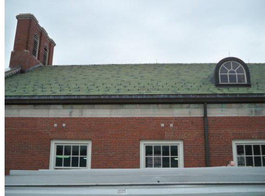
Clay tile roof
