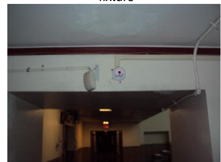
Typical motion sensor & corridor camera
