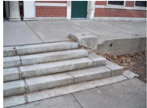
Concrete deterioration & missing railing
