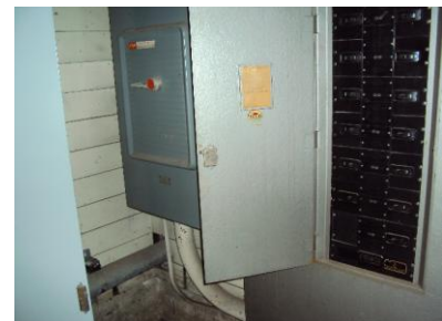
Main Distribution Panel
