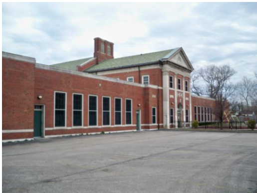
Brick requires cleaning and sealing
