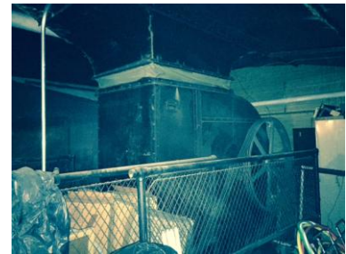
Fan Ventilation Unit with Steam Heating Coil
