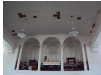
Typical Gymnasium Lighting fixture
