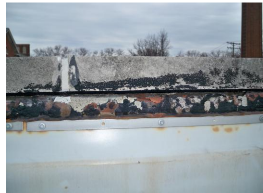
Parapet wall deterioration
