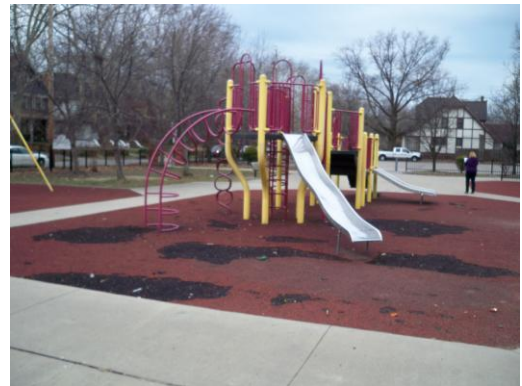
Rubber surface deteriorated
