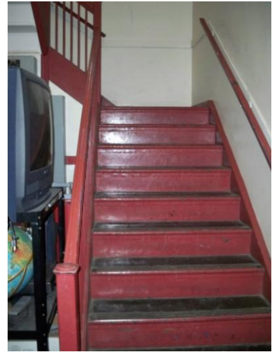
Non-compliant stair/handrail
