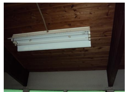
Typical Gymnasium Lighting fixture
