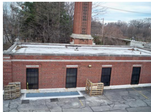
Boiler House roof
