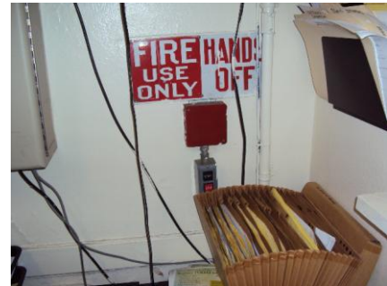
Fire alarm activation in office
