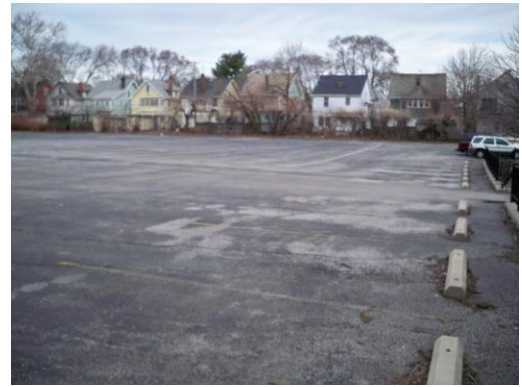
Parking lot in poor condition
