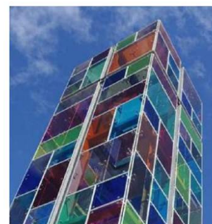
GLZ-2: BLUE LAMINATED GLASS, SAFLEX & VANCEVA COLORS PVB INTERLAYERS
