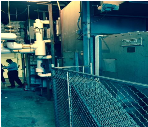
Fan Unit with Heating Coil
