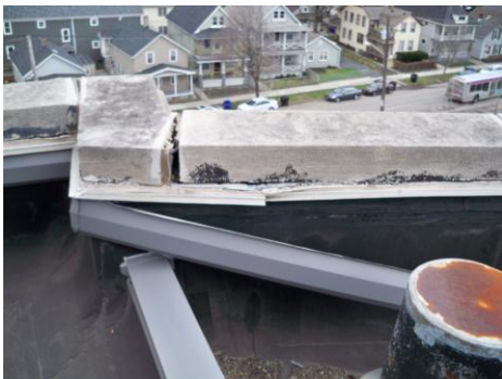
Coping joints exposed
