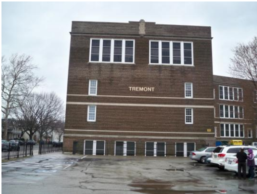
Brick requires cleaning, sealing & tuckpointing
