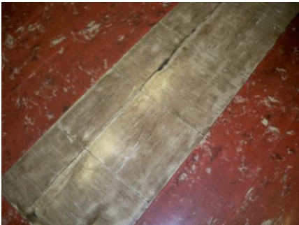
Vinyl Asbestos Floor Tiles
