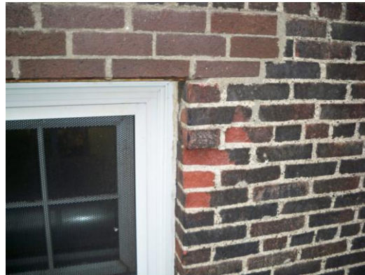
Lintels are beginning to rust
