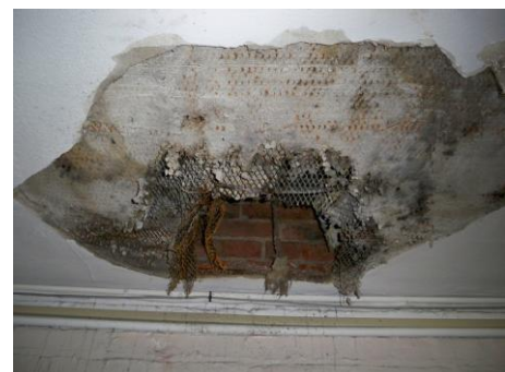
Damaged plaster ceiling
