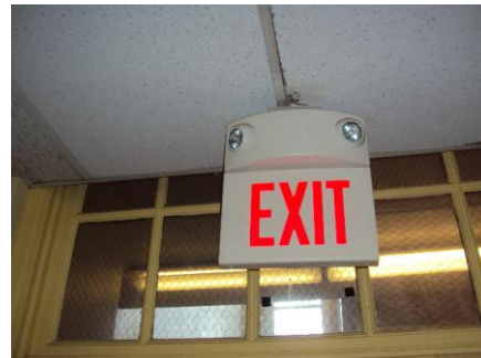
Combination exit/emergency light
