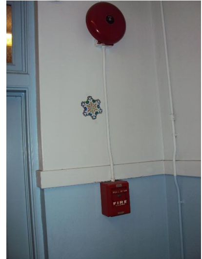
Typical pull station and indicating bell
