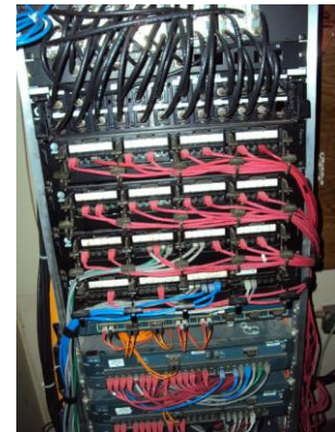
Typical technology rack on IT closet
